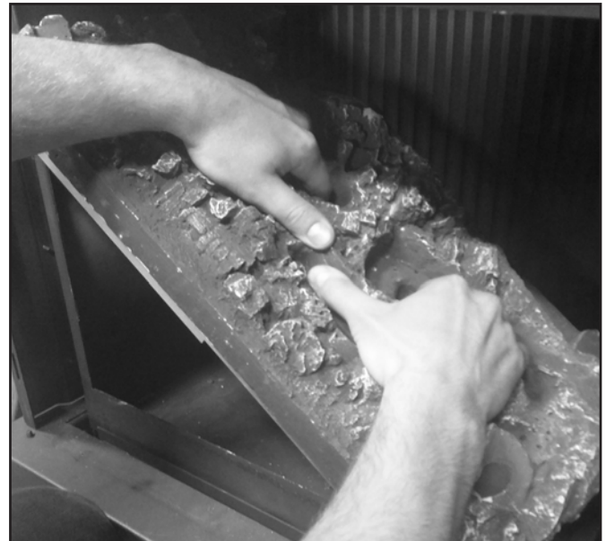
Figure 26. Burner Removal - Rotate 45 degrees
