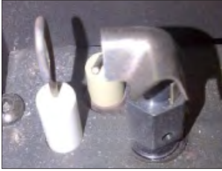
Figure 30: Proper Pilot Position.
