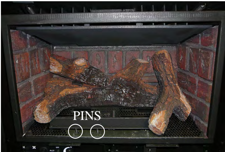
Figure 70. Third Stage Log Set Installation.
