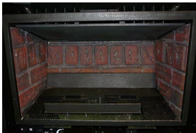
Figure 66: Side Brick Panels in Place.
