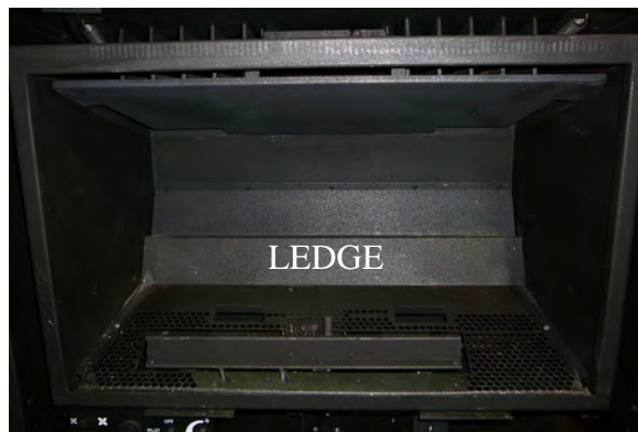
Figure 64: Back Brick Panel Ledge.
