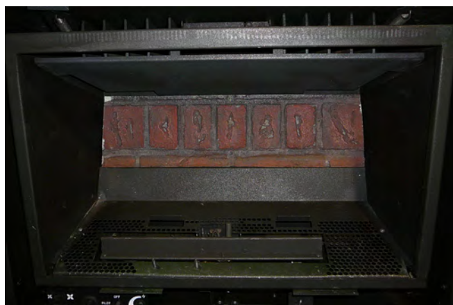
Figure 65: Back Brick Panel in Place.
