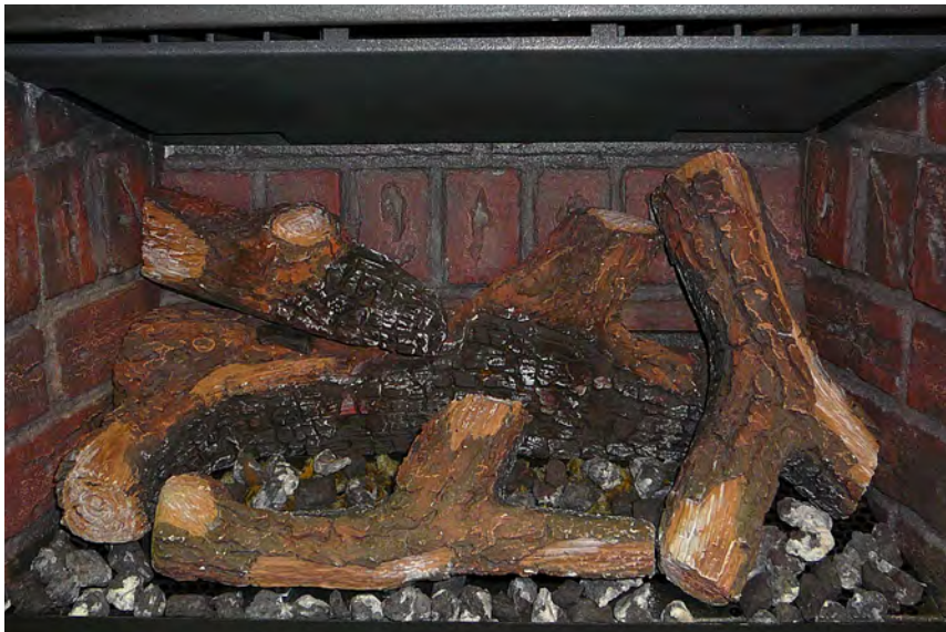
Figure 73. Log Set and Ember Installation.
