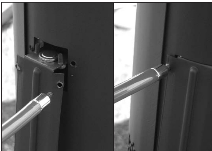
Figure 55: Spill switch installation.
