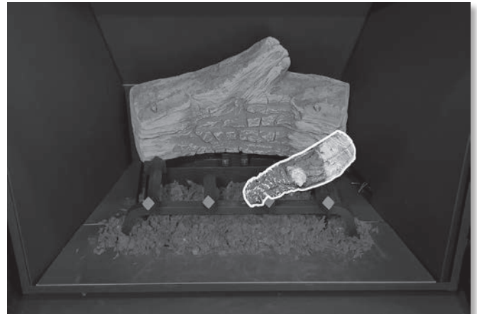
Figure 80: Log Set Installation - Step 2
