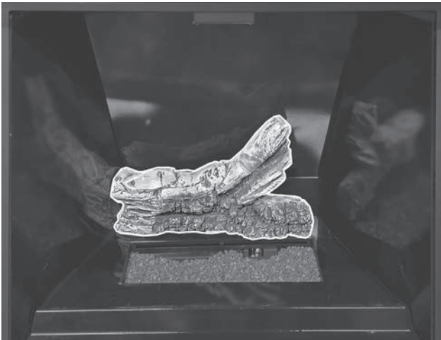
Figure 78: Log Set Installation - Step 6
