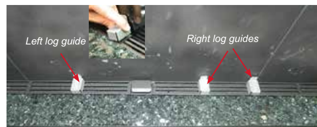
Log guides installed
