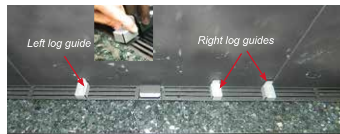
Log guides installed
