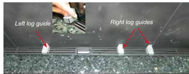
Log guides installed
