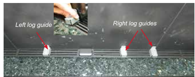
Log guides installed
