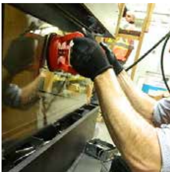
Handle glass with supplied vacuum clamps
