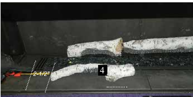
Log 4 to edge of burner
