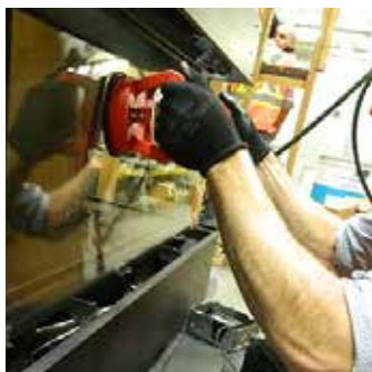
Handle glass with supplied vacuum clamps
