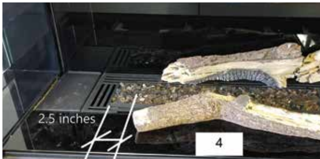
Log 4 to edge of burner
