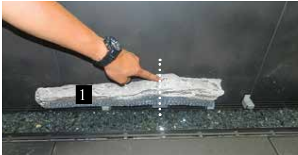
Line up knot to center of pilot hood
