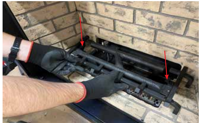
Diagram 2-Log Grate Install
