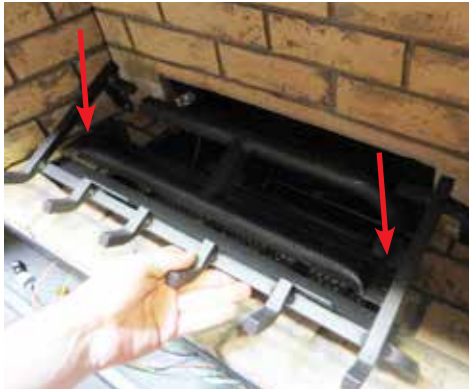
Diagram 1: Remove the left and right screws.
