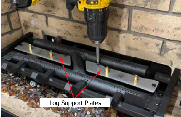
Diagram 5-Install Log support plate installation
