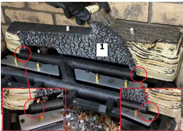
Diagram 6-Log 1 installation
