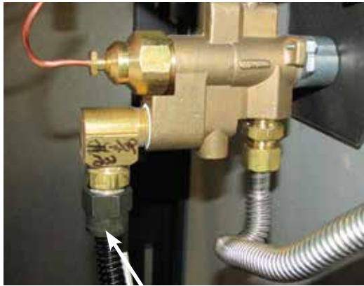
Diagram 16 Connect flex line to valve
