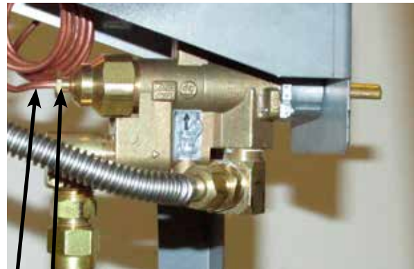
Diagram 3 Loosen nut to remove thermocouple
