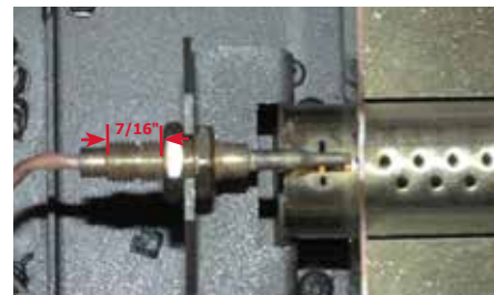
Diagram 4 Correct thermocouple placement
