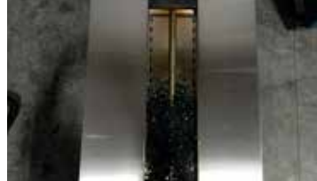
1. Start pouring Crystals/ Firebeads on one end of the burner.
